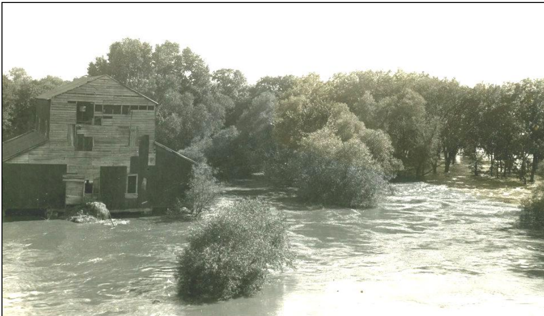
Flood on the Nemaha River at the site of old mill near Table Rock (circa 1915)
