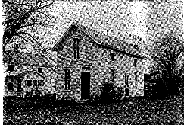
PW06-183 House: Vernacular-Gable Front
