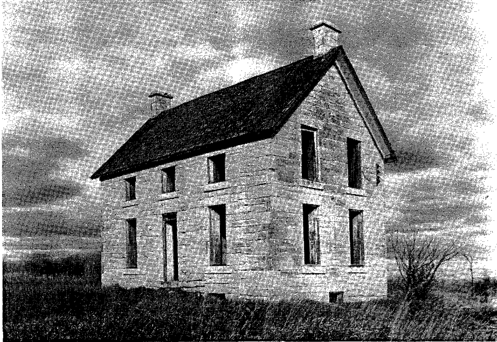
Fig. 1: Abandoned limestone farmhouse, rural Pawnee County, (PW00-006).
