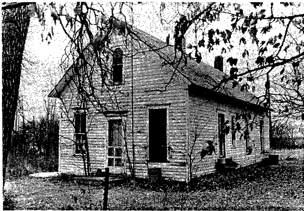
PW02-040 House: Vernacular-Gable Front
