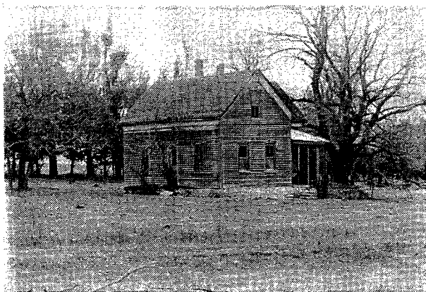
PW00-069 House: Vernacular-I House
