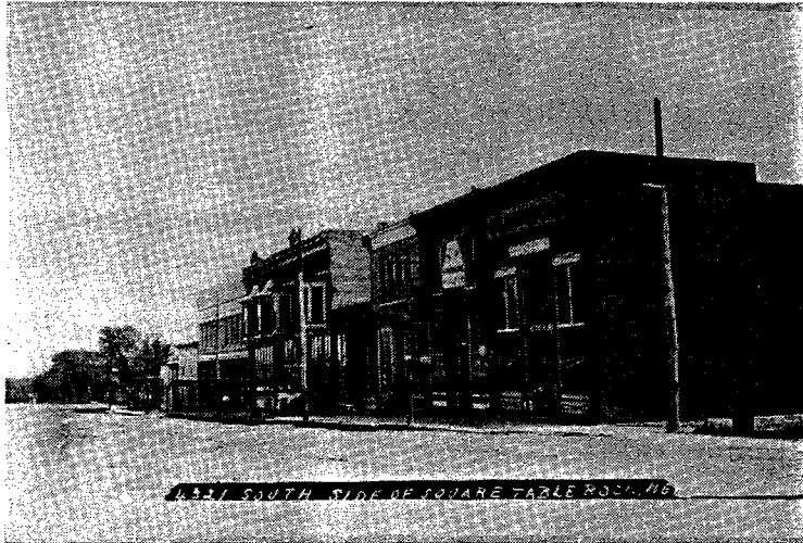
Fig. 8: South side of public square, Table Rock, destroyed by fire in 1920. (Nebraska State Historical Society Photograph Collection)
