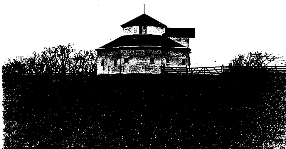
Fig. 21: Farm with Octagonal Barn north of Burchard, (PW00-035).
