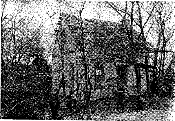
PW00-319 Abandoned Farmstead
