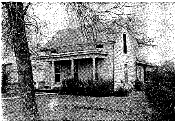
PW08-006 House: Vernacular-I House
