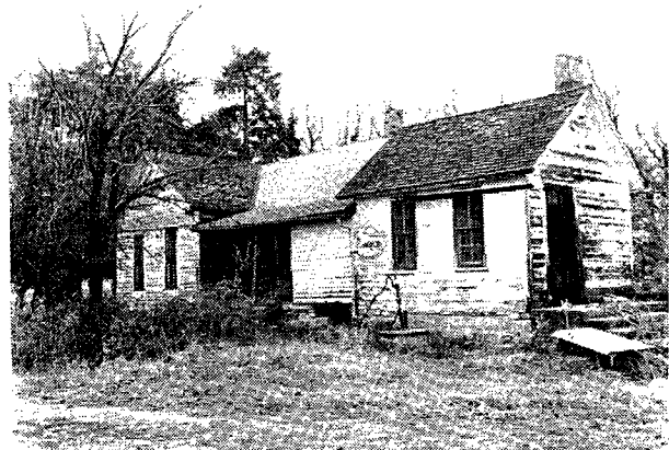
PW00-179 Wilson-Klein Abandoned Farm
