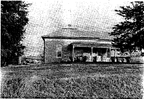
PW00-005 Limestone Farm House
