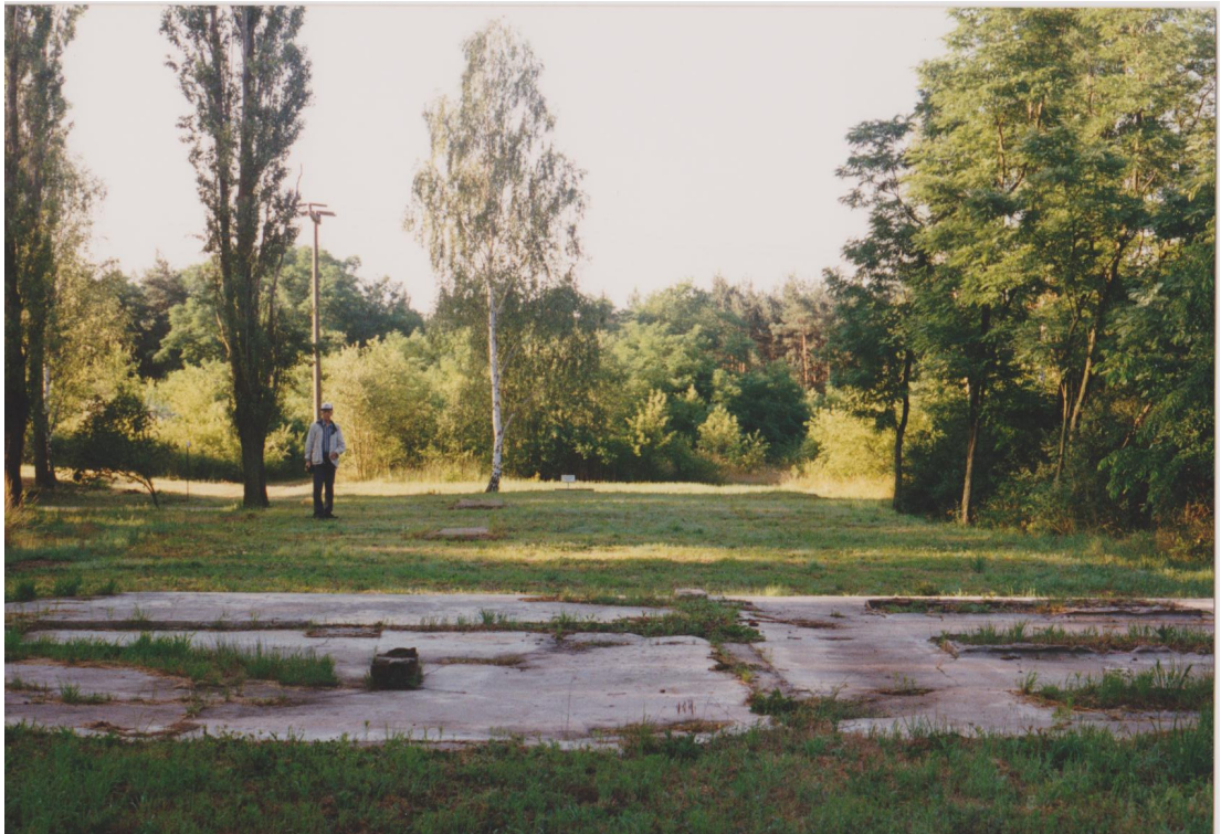
Foundations of Barracks
